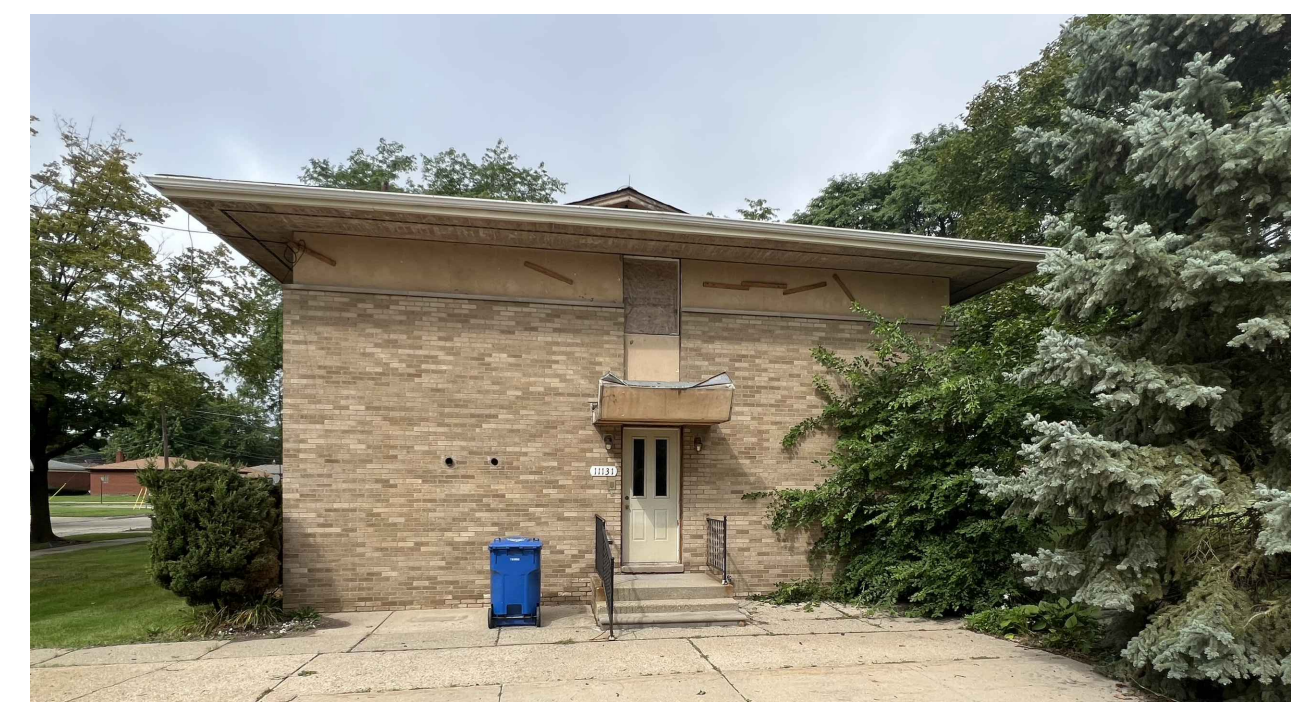
2 DEMOLITION ELEVATION AD1.0 SCALE: NOT TO SCALE PHOTO ISSUED FOR REFERENCE ONLY
