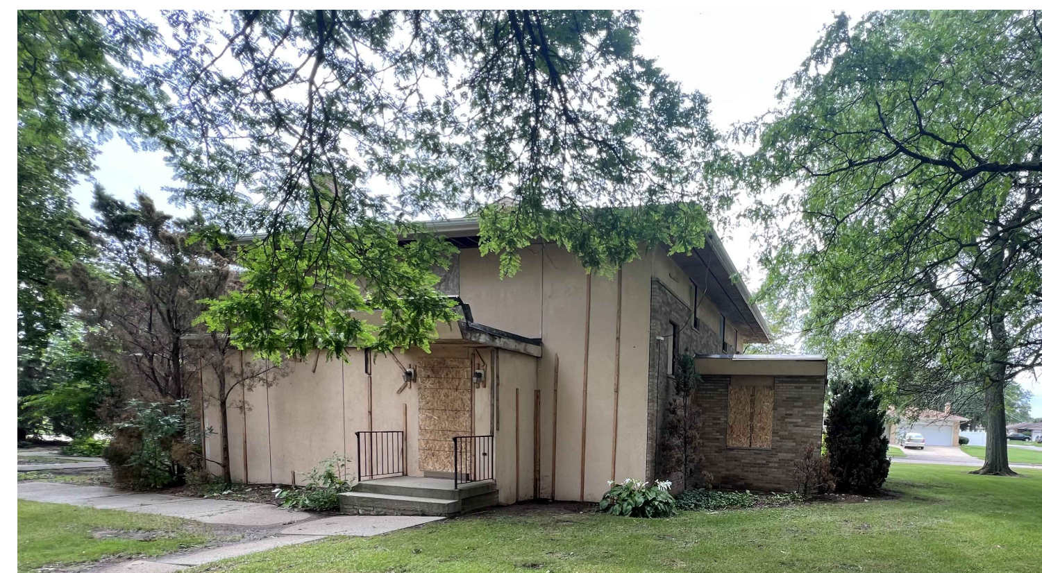
3A DEMOLITION ELEVATION AD1.0 SCALE: NOT TO SCALE PHOTO ISSUED FOR REFERENCE ONLY
